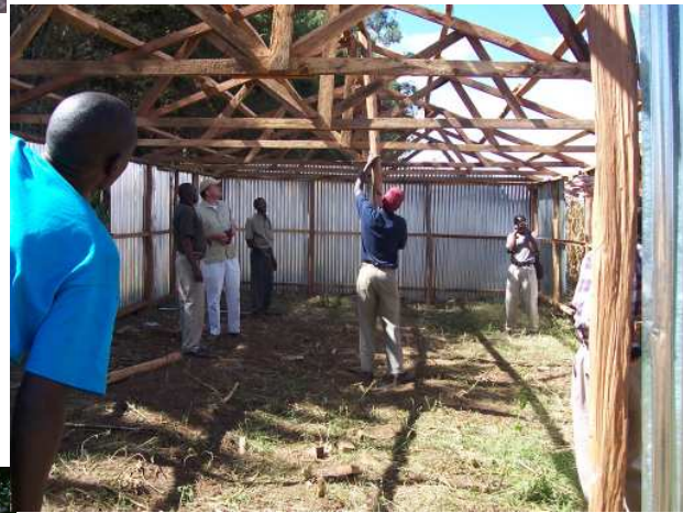
Massai new church construction
